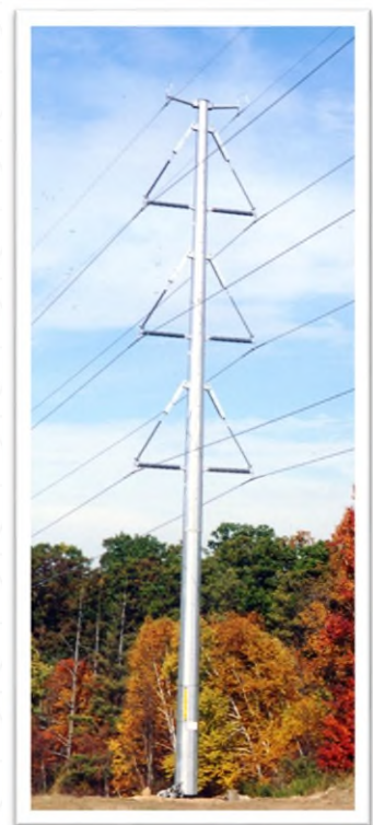
The new Brooks Industrial structures will be similar to the one shown above.
